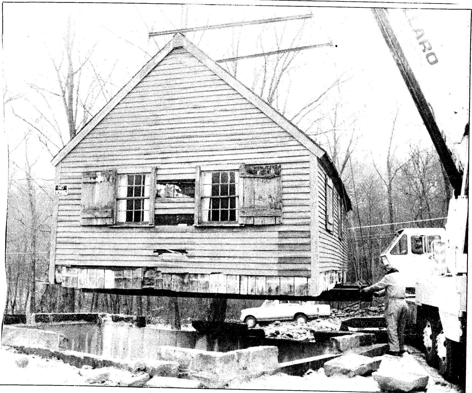
Craig Cyr of the Hebron Historical Society helps guide the Burrows Hill schoolhouse onto its new foundation Monday as the historic building was lifted off its old moorings and moved to a new and
