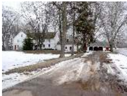
This is the John Bissell house in East Windsor off Route 5, now part of South Windsor.
